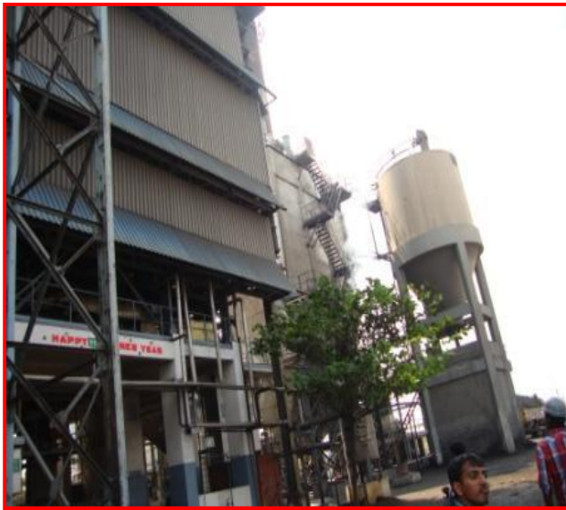
View of Power plant.
