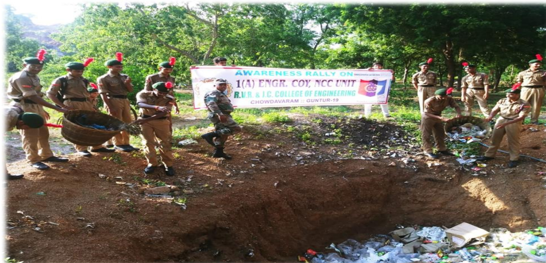
RVR & JC CE, CHOWDAVARAM – 1 (A) ENGR COY NCC, GUNTUR. 24-09-2018 CONSTRUCTING COMPOST PITS - “SWACHHATA HI SEVA”
