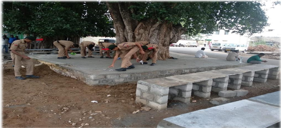
RVR & JC CE, CHOWDAVARAM – 1 (A) ENGR COY NCC, GUNTUR. 26-09-2018 CLEANING OF PUBLIC PLACES - "SWACHHATA HI SEVA"
